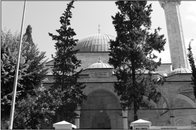
Figure 25: Bali Pasha Camii (Anthony E. Baker).
