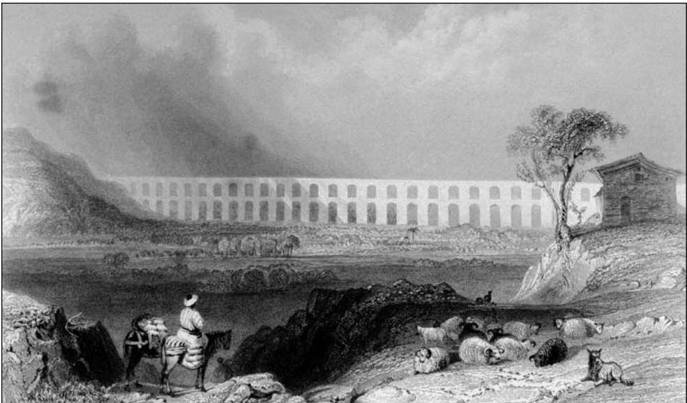
Figure 33: Uzunkemer, the Long Aqueduct (Print by Bartlett).
