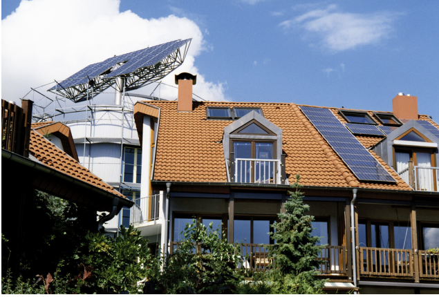
FIGURE 2.5 The Heliotrope, the Sun tracking residential house in Freiburg, Germany.
