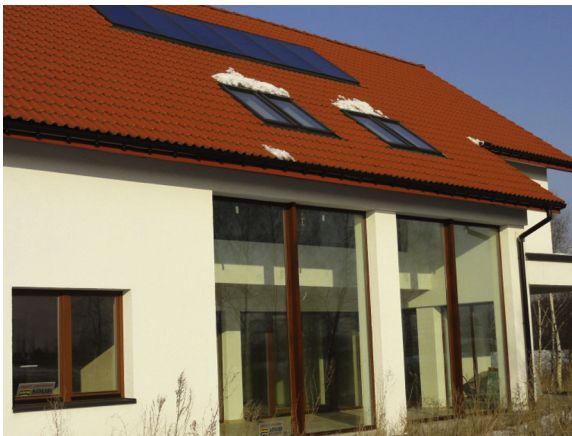
FIGURE 5.11 System with a buffer space in the form of a glazed veranda with an internal glazed partition incorporated into a building.
