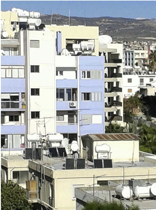
FIGURE 7.1 Thermosiphon systems in Cyprus.
