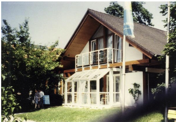
FIGURE 5.5 Typical example of a buffer space attached to a single-family house in form of a winter garden, Ulm, Germany.
