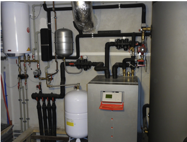
FIGURE 7.4 Solar combi heating system (indoor part, i.e., excluding solar collectors) cooperation with a ground heat pump.
