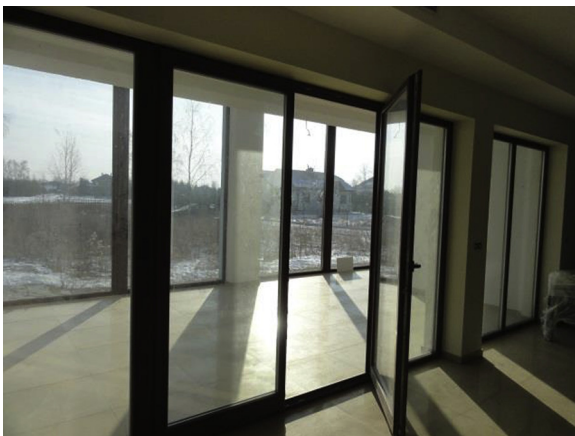
FIGURE 5.13 Buffer space seen from the inside of a single-family house.
