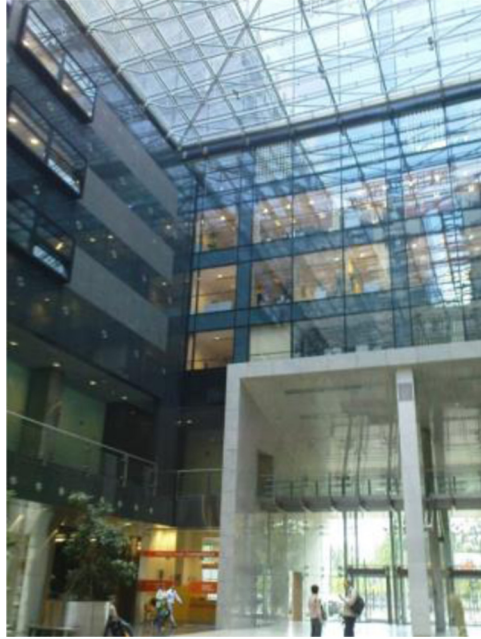
FIGURE 3.12 Horizontal glazed roof in an office building in Warsaw, Poland.
