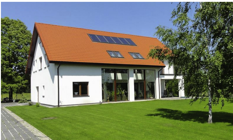
FIGURE 5.7 Example of a buffer space incorporated into the structure of a single-family house, Warsaw, Poland.
